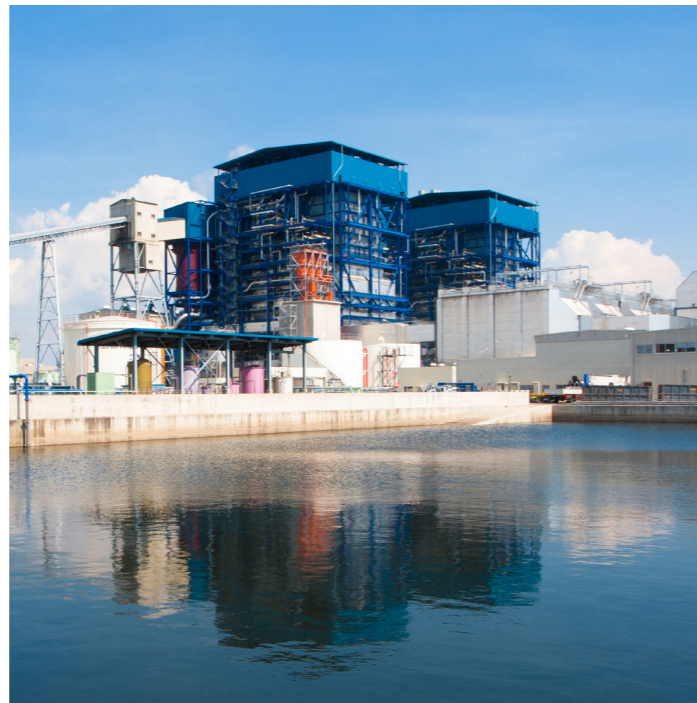
WASTE WATER TREATMENT
