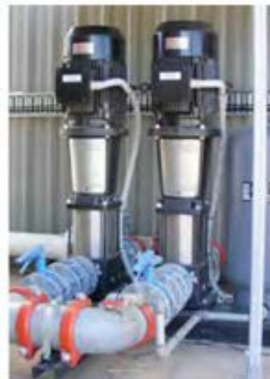
On-Site Installation, testing and commissioning
