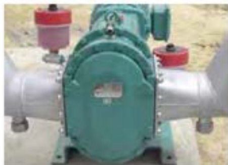
Feed pump for substrate in a biogas plant. Flowrate up to 40 m 3 /h at pressures up to 2 bar.
