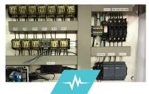
UL CSA listed electrical and instrumentation control panels, VFD and PLC driven panels, or Variable Speed Drive (VSD) panels to control and minimize transient pressures.
