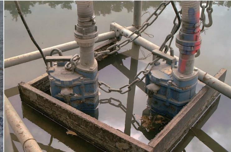
**KTV:** Drainage pumps of lightweight compact design
