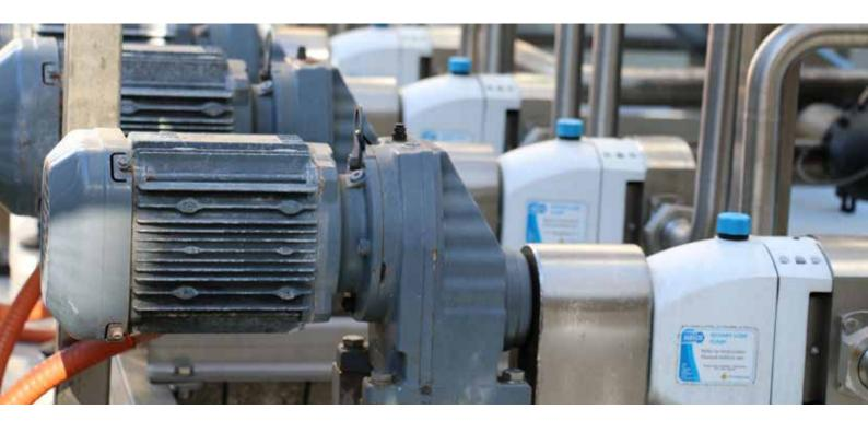
**Gear Pumps** Rotary Gear Pumps consist of at least one or two sets of rotating gears with intermeshing teeth. As the teeth separate, they create a partial vacuum which is filled by the fluid. When the gears continue to rotate, the fluid becomes trapped and carried around the casing to the discharge port of the pump. Gear pumps can be external or internal.
