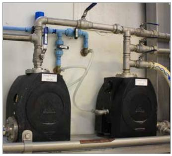
The plastic solid-body construction of Almatec® E-Series AODD Pumps eliminates the small crevices or cavities that can be found in injection-molded models. It is in these crevices that liquids can accumulate and leak paths can be created.
