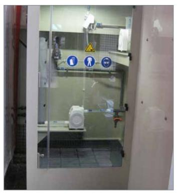
Harsh chemicals can cause compatibility concerns when used with some types of pumps. Almatec<sup>\*</sup> E-Series AODD Pumps can be constructed of plastic materials that are specifically compatible with the chemicals that are being handled, which eliminates corrosion and leak fears.
