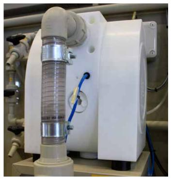
During their operation, injection-molded AODD Pumps can bounce, which can loosen pipework and increase the chances of a chemical leak. Almatec<sup>\*</sup> solid-body AODD Pumps are more stable during their operation, which leads to a higher level of product containment.
