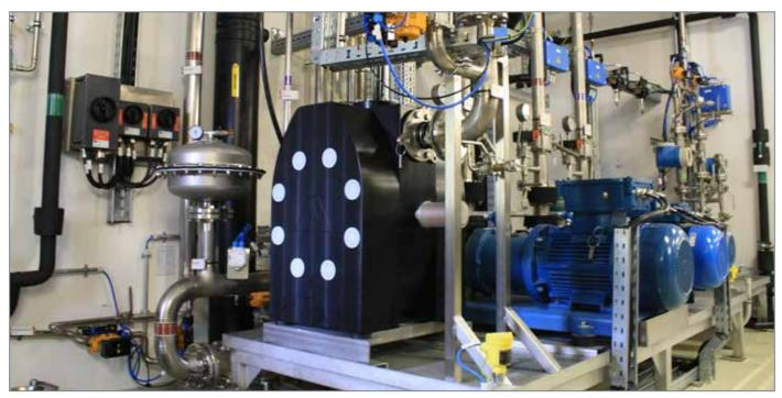
The need to use hazardous or dangerous chemicals in the manufacture of numerous products or the completion of a wide array of industrial processes is a fact of life. Utilizing Almatec<sup>\*</sup> plastic solidbody E-Series Air-Operated Double-Diaphragm (AODD) Pumps will help ensure that these liquids are fully contained and that their release will not harm humans, animals or the environment.
